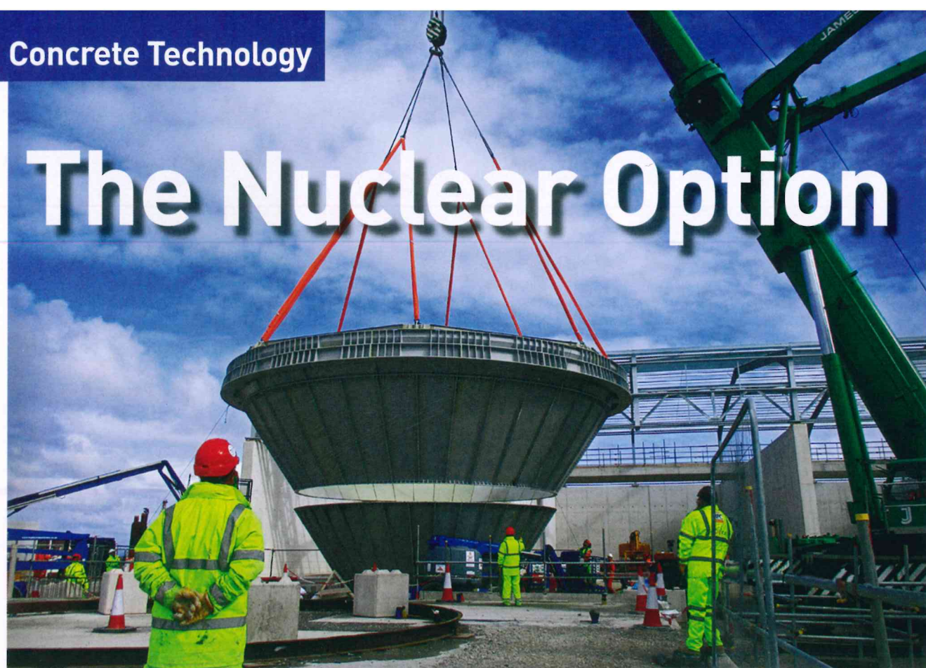
Construction of the base cone for the ground granulated blast-furnace slag (ggbs) silo (April 2017)
