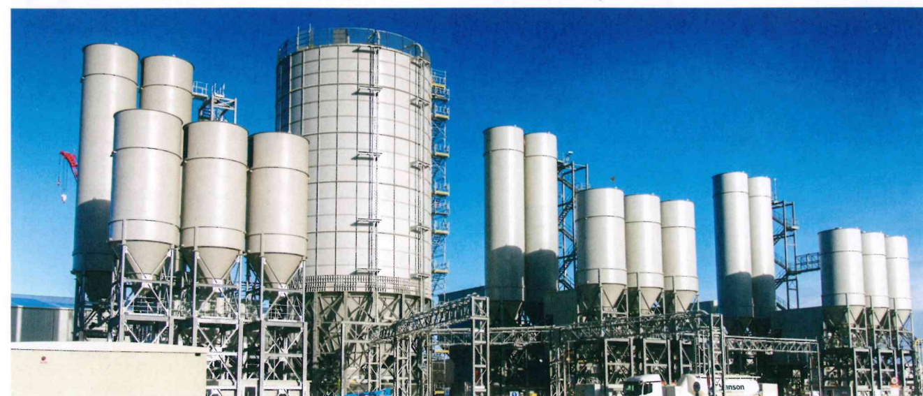
View of Bylor's three concrete batching plants, including the ground granulated blast-furnace slag (ggbs) silo, at Hinkley Point C (December 2017). Image: EDF Energy
